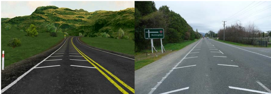
Figure 5. A herringbone lines perceptual countermeasure as applied in simulation (left) and on SH57 in Levin, NZ (right).
