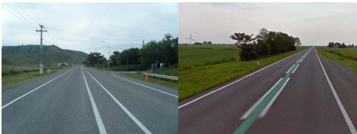
Figure 7. Possible road treatments for hazardous rural roads; a rural median trial in New Zealand (left) and The Netherlands (right).
