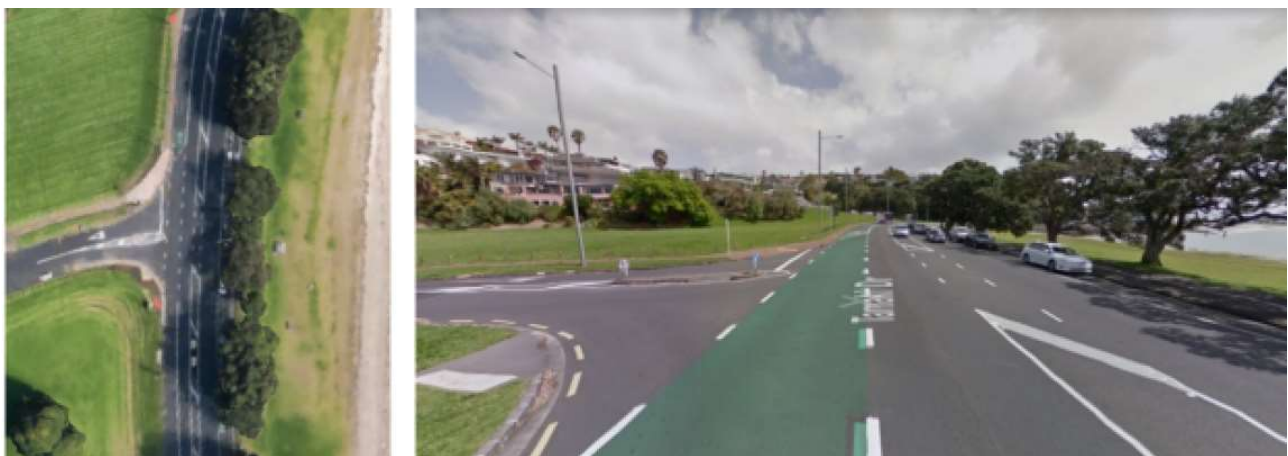
Figure 5: Site 2 intersection between Tamaki Drive and Watene Crescent
