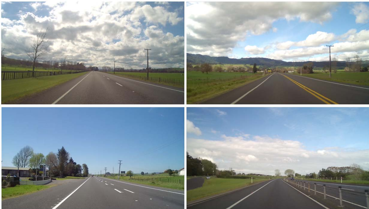
Figure 1. The four median treatments selected for testing. Clockwise from top left: Dashed white control, double yellow, wire rope barrier, wide centreline.
