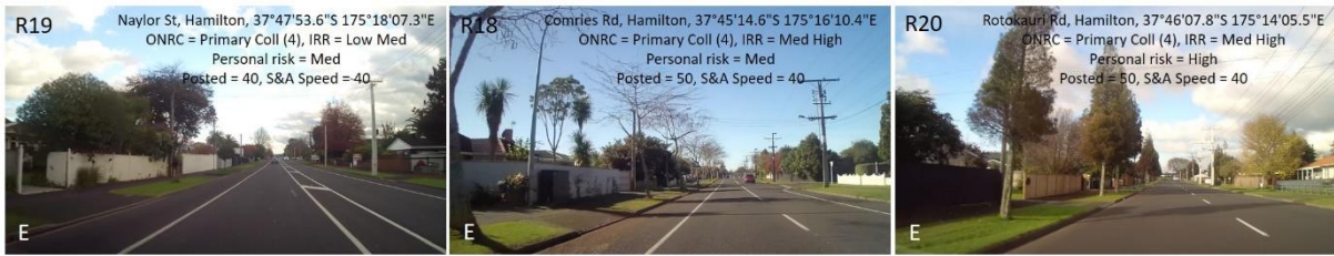
Figure 15. Roads classified as ONRC 4 (Primary Collectors) with poor speed limit credibility (R19, left hand side) and good speed limit credibility (R18 and R20). The letter in the bottom left corner indicates the participants' sort category.
