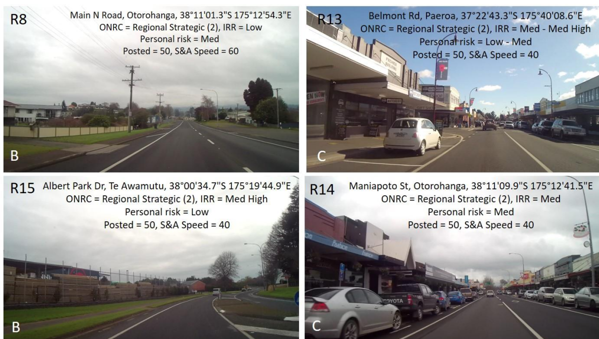
Figure 13. Roads classified as ONRC 2 (Regional Strategic) with poor speed limit credibility (R8, R15, left hand side) and good speed limit credibility (R13, R14, right hand side). The letter in the bottom left corner indicates the participants' sort category.
