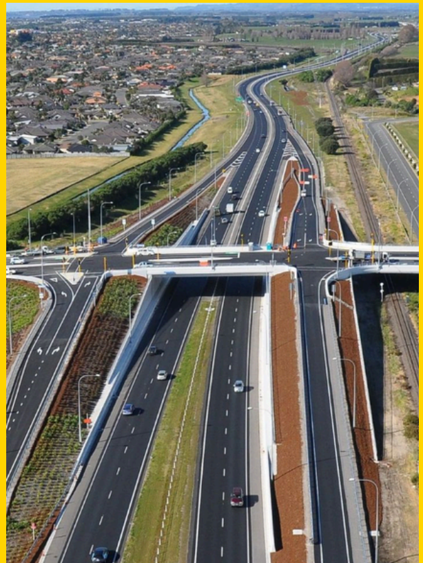
The building of the Tauranga Eastern Link highway has helped see a 50% reduction in fatal and serious crashes on SH2 from Mount Maunganui to Paengaroa. Image: NZTA
