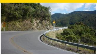
Easing of three particularly tight corners on the Hill Rd is needed to enable large trucks to negotiate them without crossing the centre line.
