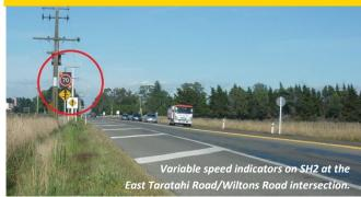
Variable speed indicators were installed at the East Taratahi Road/Wiltons Road intersection in 2016. They have improved safe access to SH2 with no accidents recorded since the signs were erected.
